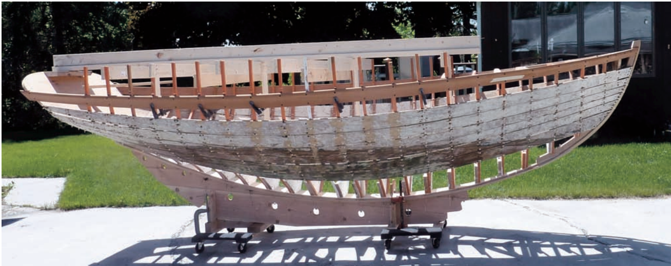
Figure 1 – A view of the sheer after the author made corrections. The beam hovering over the boat maintains the centerline of the boat down the actual center. The beam is attached to the cross members at the remaining molds.
