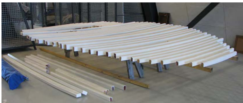
59) Prefabricated deck beams, October 2010. (Pedrick)
