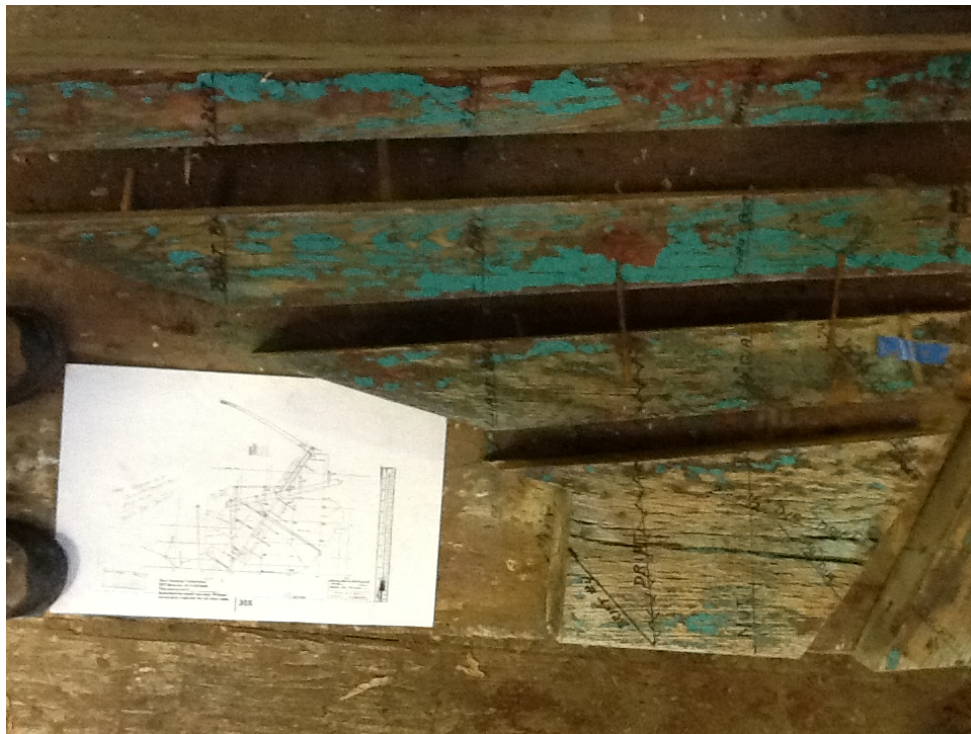
Figure 5 Deadwood and drawing. Discrepancies were noted, but deadwood was reassembled “as built”
