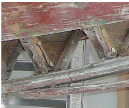
Figure 35 Rotted frames bottoms at #8 & #7.
