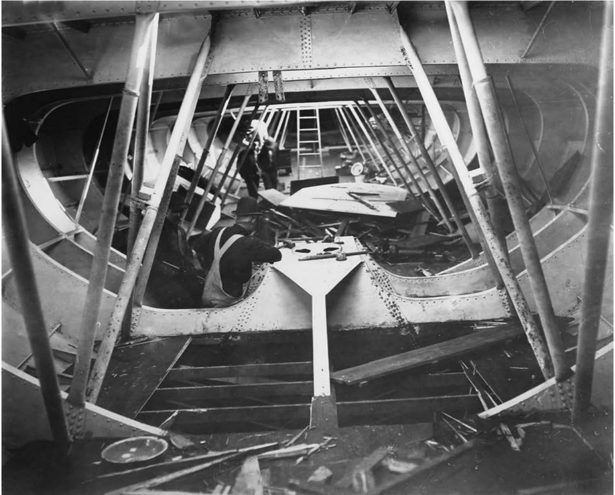
Exhibit 11: RELIANCE below deck looking forward with the mast step in the foreground showing diagonal bracing and web-frame with flanges (bulbs) and angle fasteners to hull and deck. Source: Herreshoff Marine Museum Archives. Photographer unknown.
