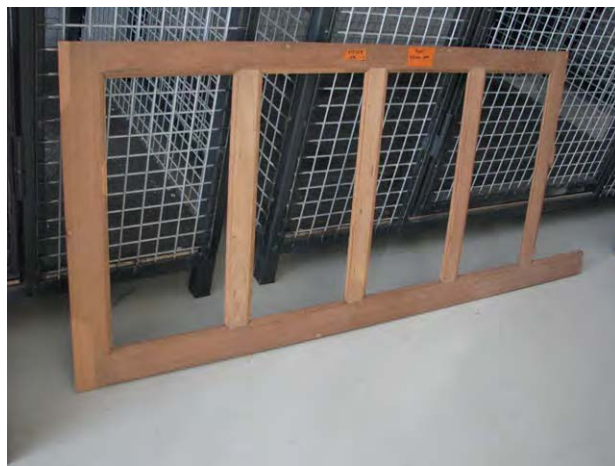
68) Stiles and rails of a set of fielded panels, which have been removed to be restored separately. This piece was reduced in size to fit outboard of the new pilot berths. (Pedrick)
