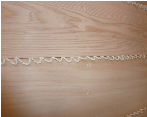
Figure 30 Looping in the cotton wicking. This is called “stitching” the seam.
