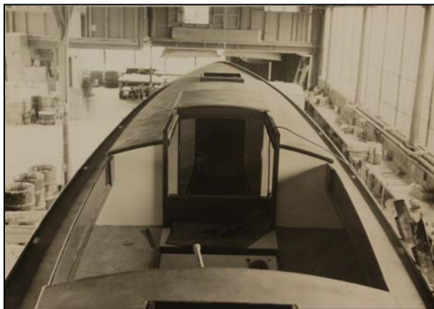
8.) Deck and cockpit fitted at the Anchorage shops (© courtesy The Anchorage, Inc. – Dyer Boats).
