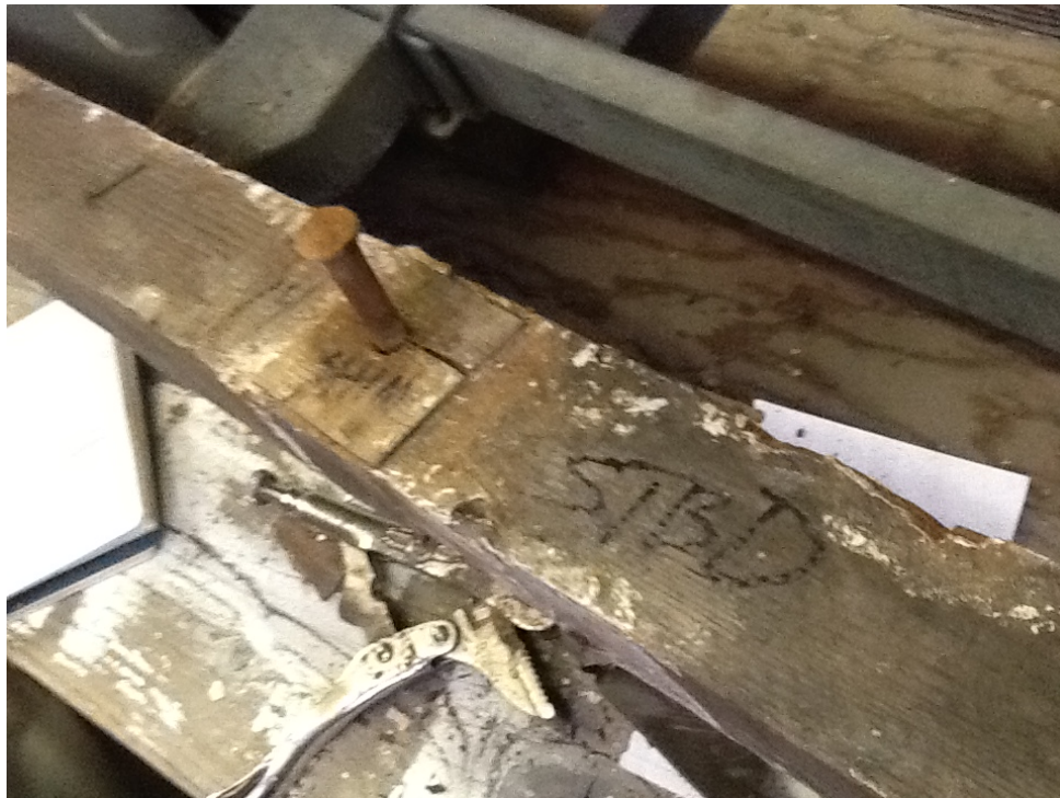
Figure 6 Shear clamp showing shim that was placed under the deck beam prior to bolting. The same shim will be reinstalled.
