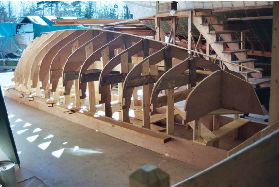
Fig. – 6 Strongback and Mold Setup Before Adding Boat Components
