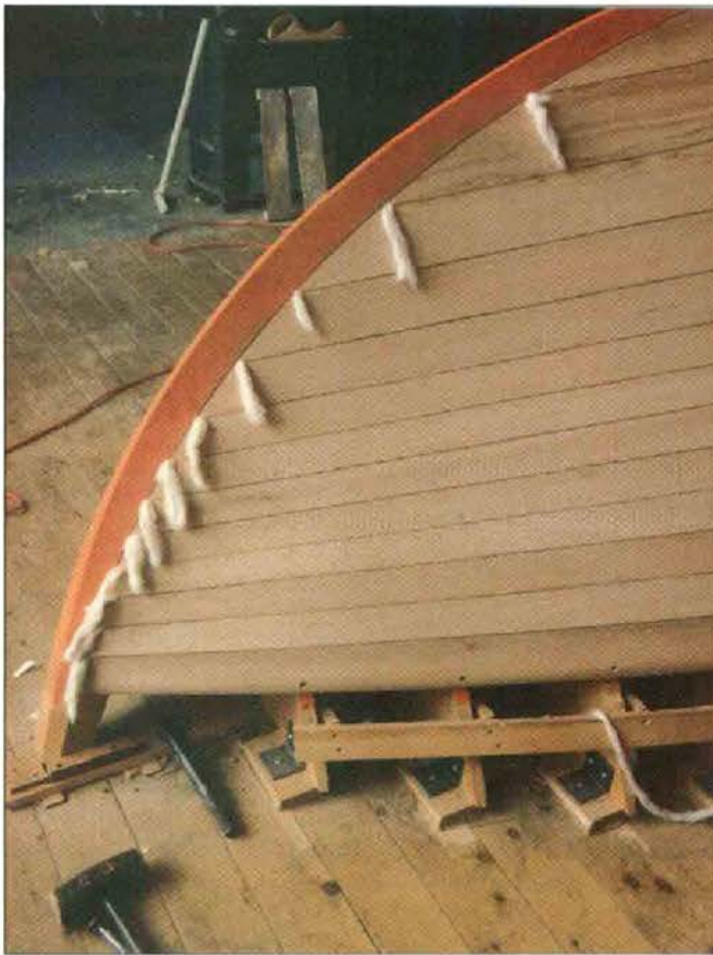
11 We used Atlantic white cedar throughout the hull in lieu of cypress garboards and Port Orford cedar planking. In time-honored fashion, the seams are caulked with cotton, and painted and payed.
