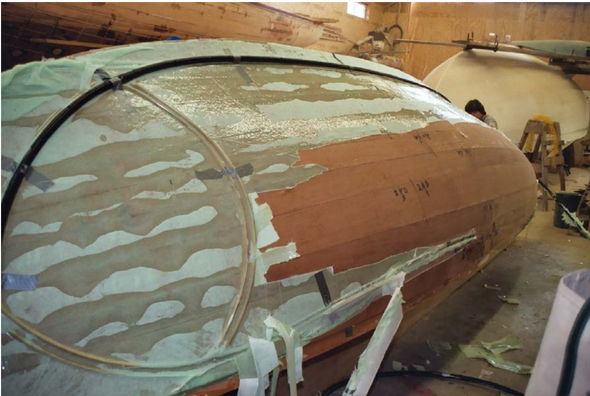
Fig. – 14 Hull Fabrication – Peel Ply and Excess Glue Removal
