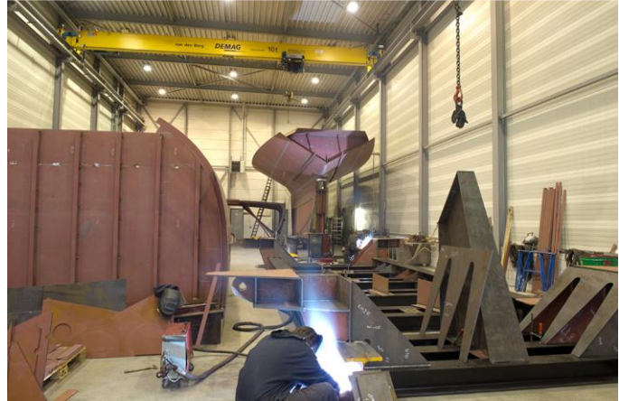
Figure 2 –2012 INGOMAR Under construction in Holland
