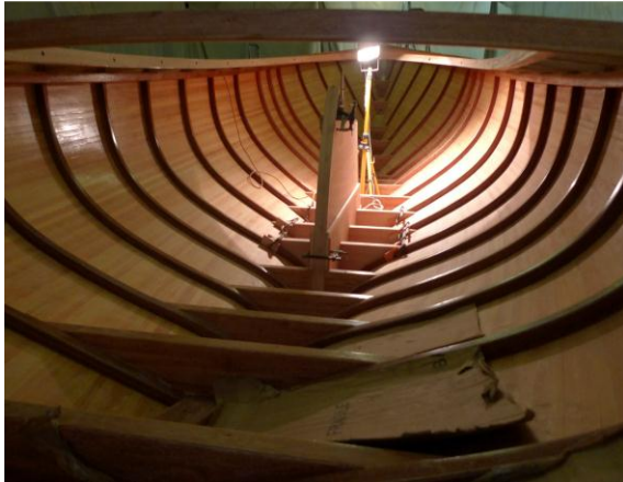
Figure 1 – Internal framing and planking
