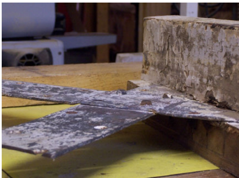
Figure 2 – June '07 – Crossing of Original Steel Deck Diagonal Straps.
