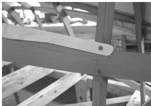
Detail of battens ending into the chine.
