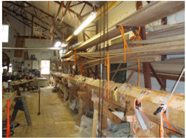
Figure 3- After glue up. Mast still in clamps.
