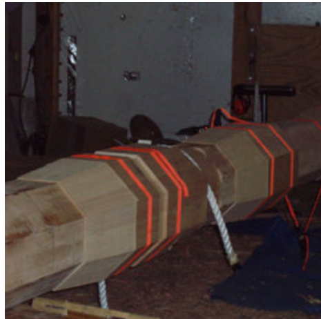
Figure 4- Continuous bolsters or cheeks around mast to support rigging.
