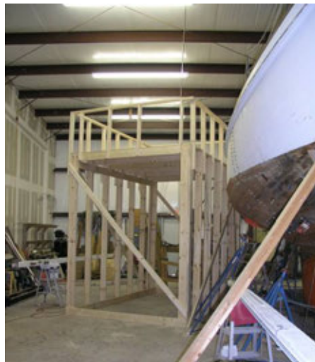
Figure 38 - Deck-level work platform.
