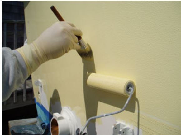
Figure 3 - Rolling & tipping using the “Gang” painting method.
