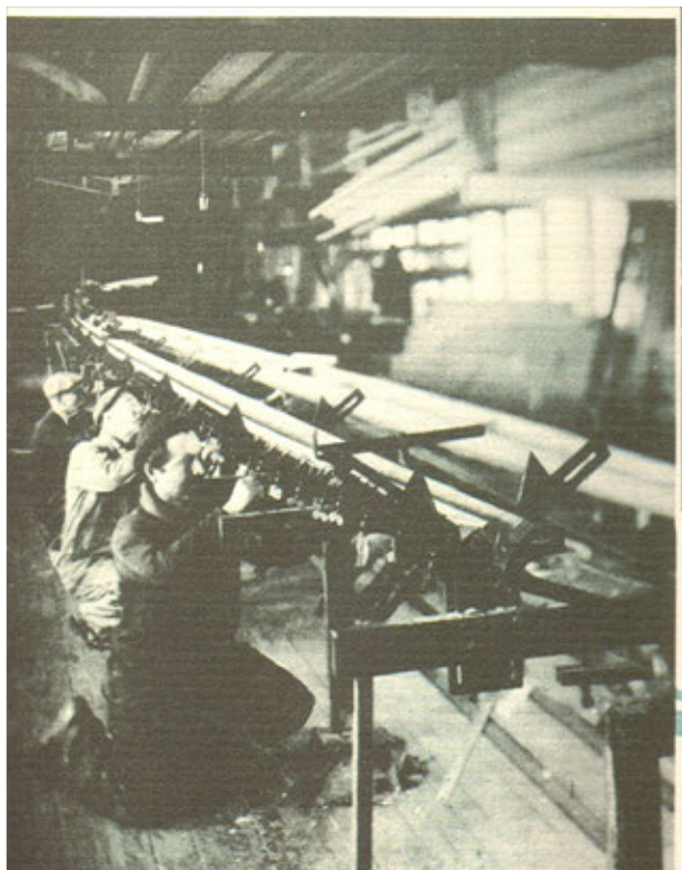
Figure 3 - Spar glue-up at the Herreshoff Manufacturing Company.
