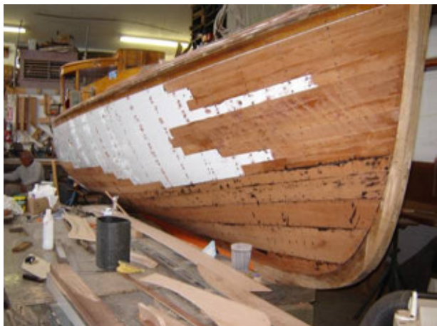
Figure 14 – New planking scarfed and butted to existing white planks.
